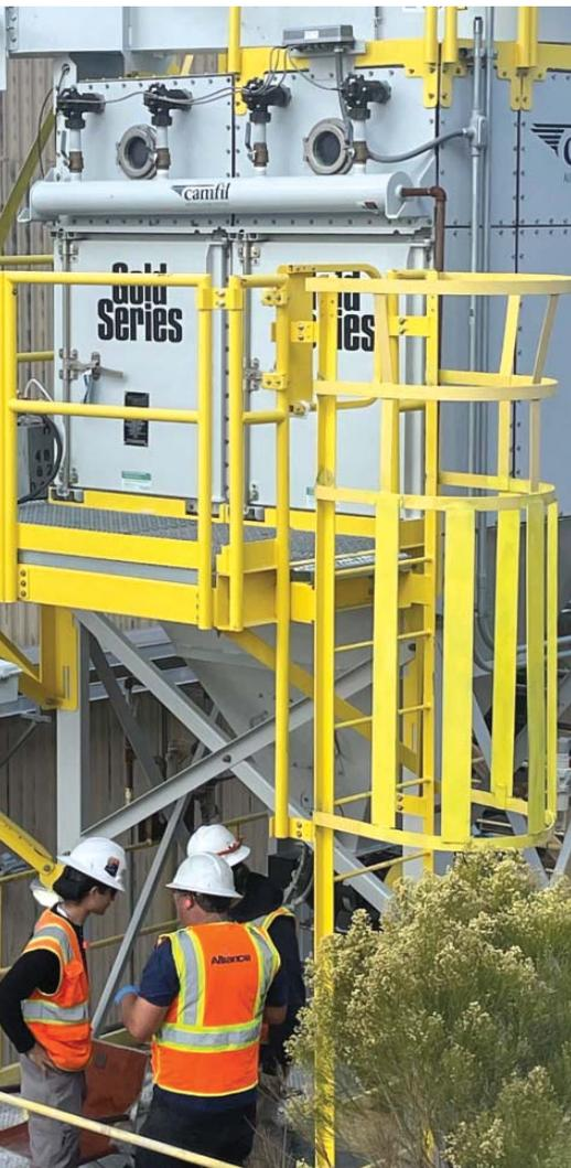
The mine realized 20 gpm in water savings by replacing old wet scrubbers with new, water-free dust collectors. (Photo: Capstone Copper)
