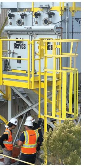
The mine realized 20 gpm in water savings by replacing old wet scrubbers with new, water-free dust collectors. (Photo: Capstone Copper)
