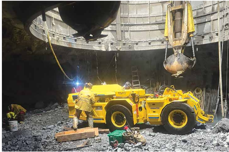
An LHD arrives at the shaft's first level to begin lateral development. (Photo: Hermosa)
